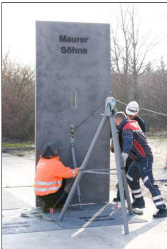
MMBS unit being secured with locking prop
