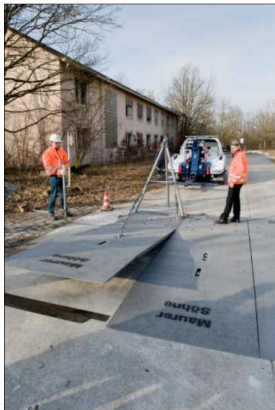
MMBS unit being raised by a truck mounted winch
